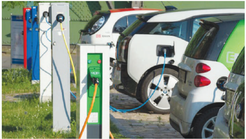
A picture showing electric vehicles connected to chargers
